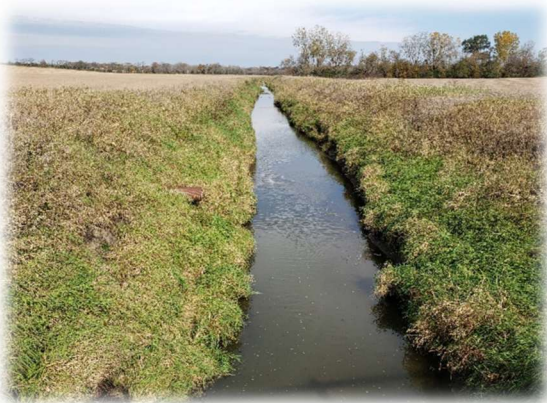
Low Flow Condition 3 Mile Road Looking North
