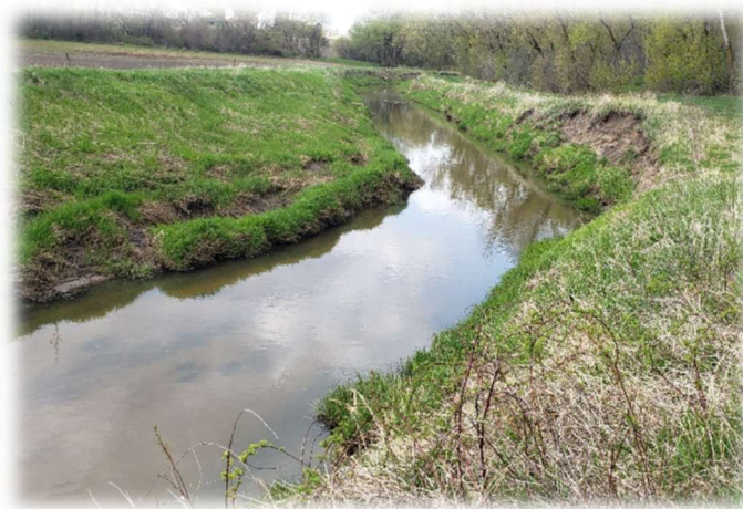
Deposits on the Inside and Scouring on the Outside
