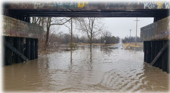
Flooding at 67 th Drive
