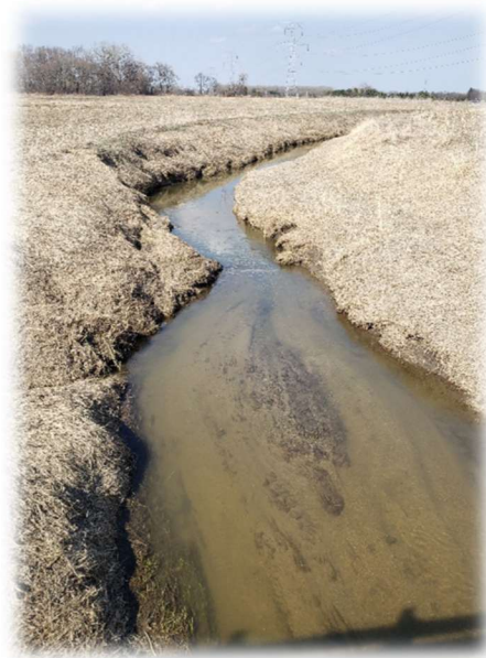
Accumulated Sediment at CTH A
