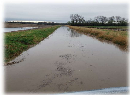
High Flow Condition 3 Mile Road Looking North
